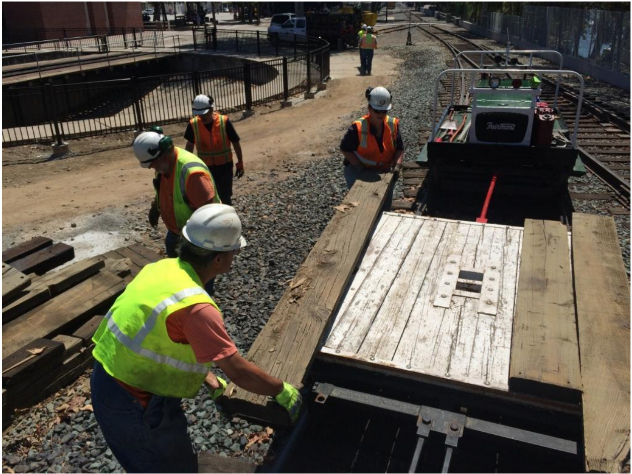
John and Heather load old turntable planks on the flatcar
