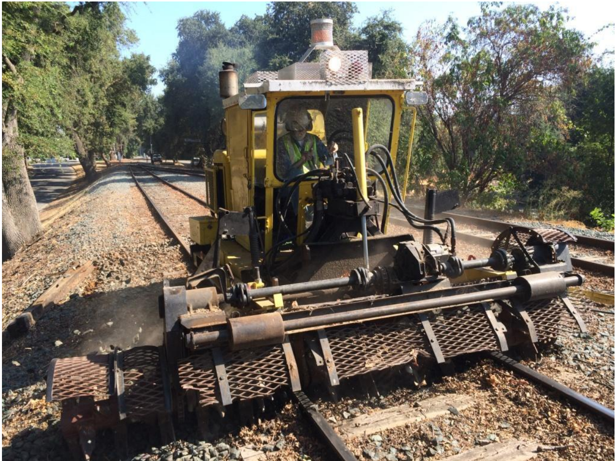
Having the scarifer on site saved us from having to dig out all the cribs by hand. It's an amazing machine
