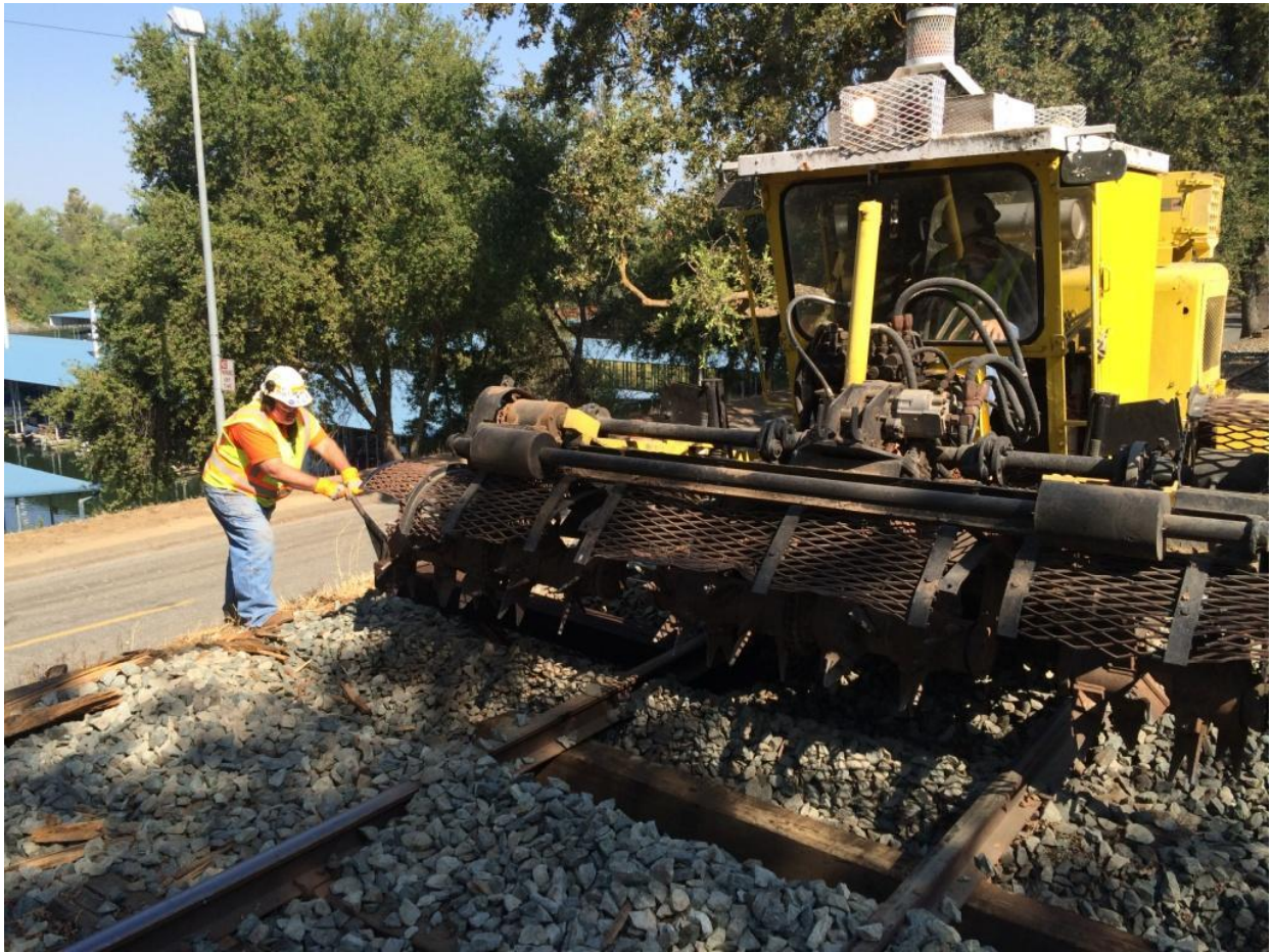
Mike F. guides a tie into place
