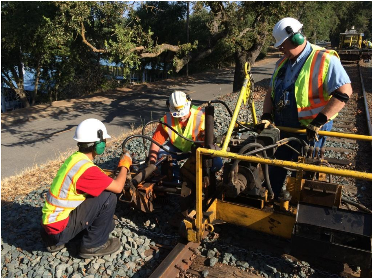
Josh, Mike F., and Chris have to use the chains to pull out a splintering tie
